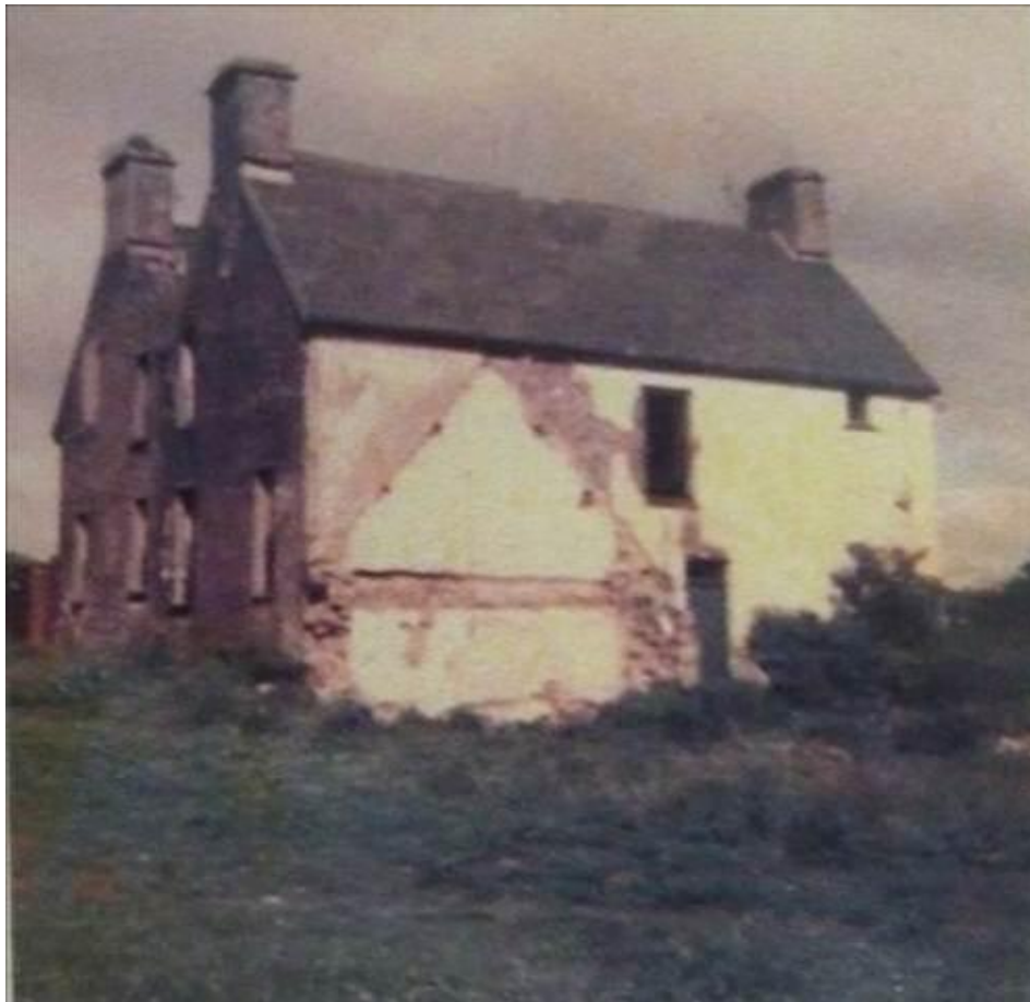
Photo 2: Eastern facade of Machynys Farm following demolition of former attached barn c.1970 (CRO ref: DX/35/2)
