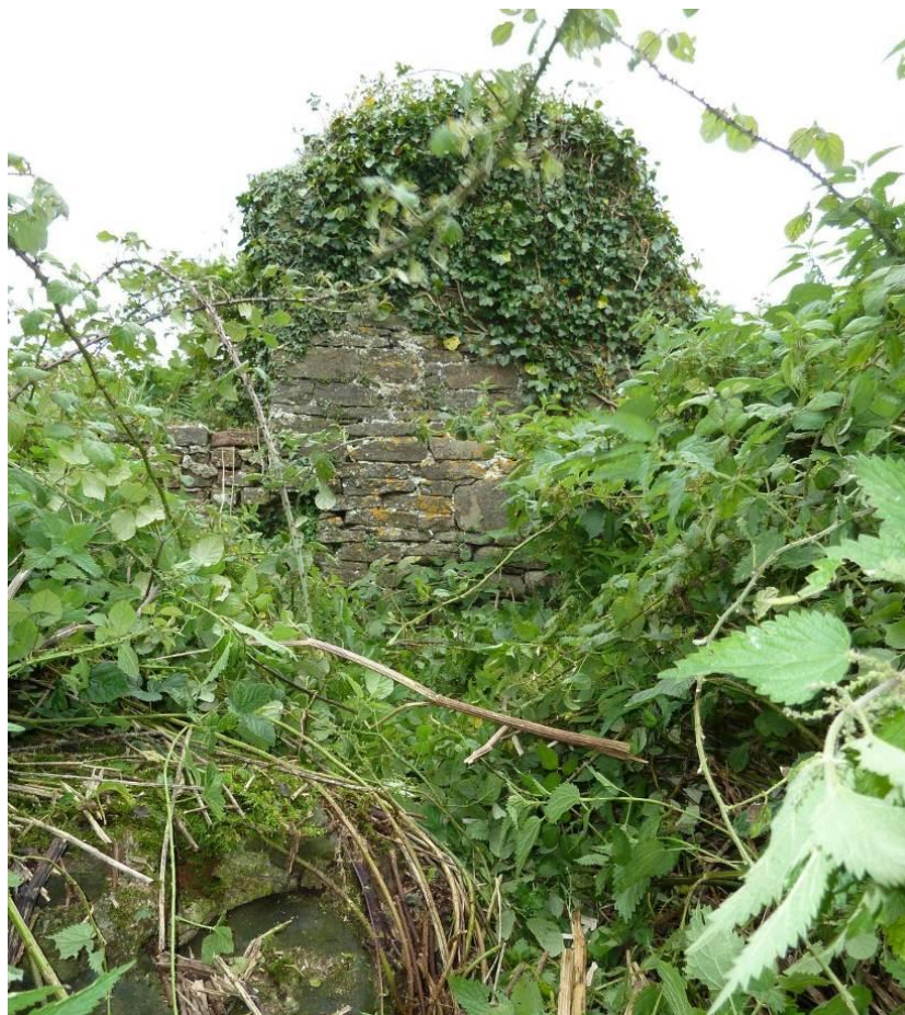
Photo 8: A segment of mortared building wall.
