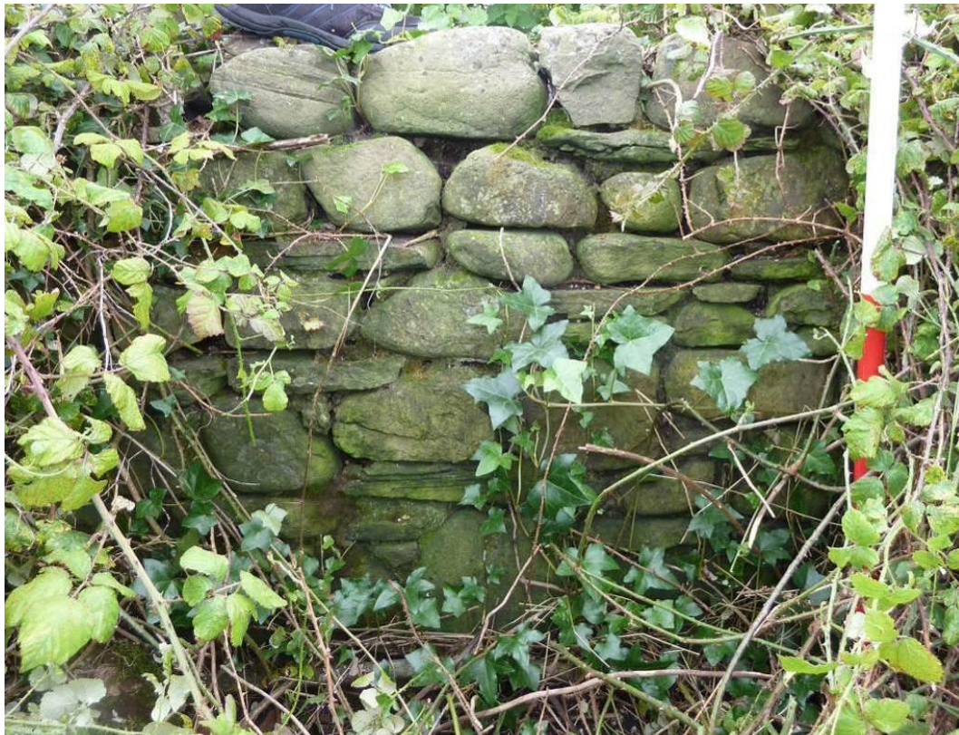
Photo 9: Further section of garden/enclosure wall.
