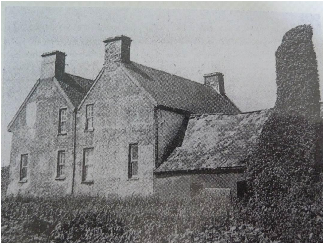
Photo 5: Southern façade of Machynys farmhouse taken in the 1960s, showing the double-pile construction of the main house with the eastern wing and an ivy-clad external lateral chimney stack (with possible arch visible in ivy)
